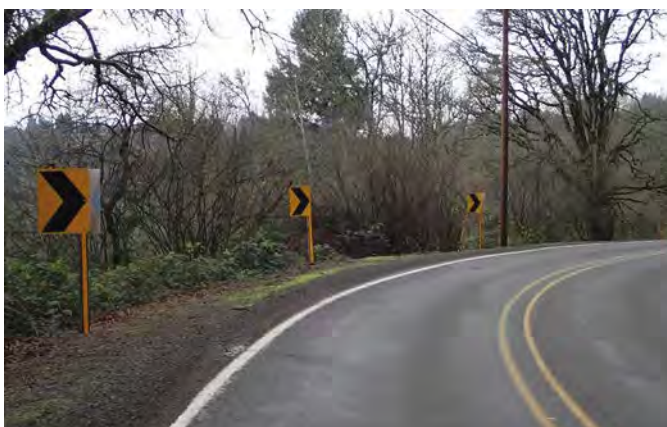
(Photograph provided by Federal Highway Administration)
