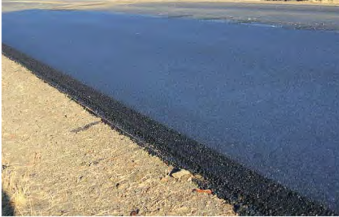
(Photograph provided by Texas A&M Transportation Institute)
