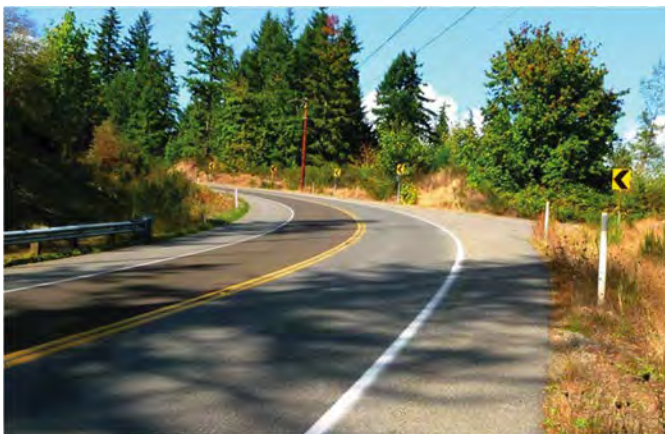
Figure 6. HFST application (left lane) with original pavement (right lane).
