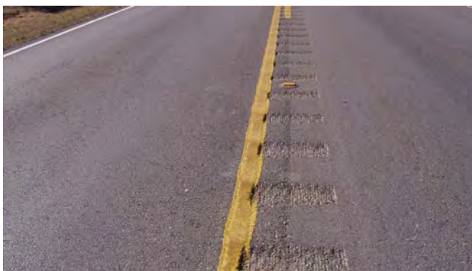
(Photograph provided by Texas A&M Transportation Institute)
